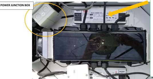
DATA CABLES CAN PASS DIRECTLY INTO BOB POD SEALED AREA VIA PORTS PRE-INSTALLED ON COOLER BOX AS SHOW.
