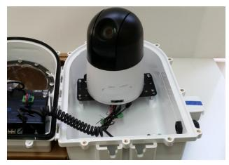
Snap the Sony SNC-WR630 Camera on Ceiling unit and Secure into D2; Complete with proper power & Ethernet wiring to
