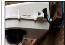
Make sure to create a “U” shape drip loop with the cables to prevent water from pooling and possibly seeping inside.
