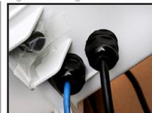
Make sure to have only one cable per gland and tighten them really shut to completely seal D2 enclosure from the outside.
