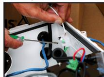
Have a qualified electrician connect an external power source to D2 terminal power block. See manual for more details.
