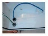
Push plug into conduit mouth with finger tips till it flush with outside of fitting.
