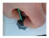
Pinch Plug to compress over wire, and insert into conduit feed mouth.
