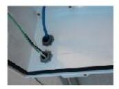
1) Pull wires to final installed length.
