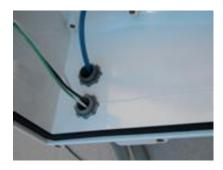
1) Pull wires to final installed length.
