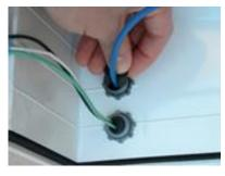
4) Push plug into conduit mouth with finger tips till it flush with outside of fitting.
