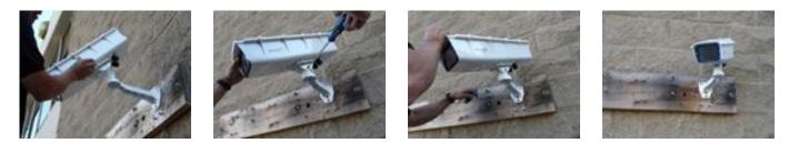
Using two side screws removed in first step, re-assemble Tilt bracket to wall mount as shown. Loosen & then re-tighten screws for Pan & Tilt adjustment to arrange housing to desired viewing angle. Securely tighten all fasteners to final position. Install Power and Data cables as desired thru ports on rear of S-Type enclosure. Always create a "drip-loop" for wire or cable that comes from above enclosure.
