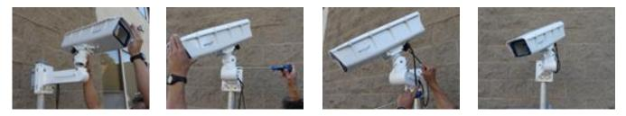
Attach housing to arm as shown, tighten screws evenly but firmly on both sides of housing. Adjust housing to desired position using both pan & tilt adjustment fasteners and tighten all bolts evenly & securely, so housing is pointing into final position.
